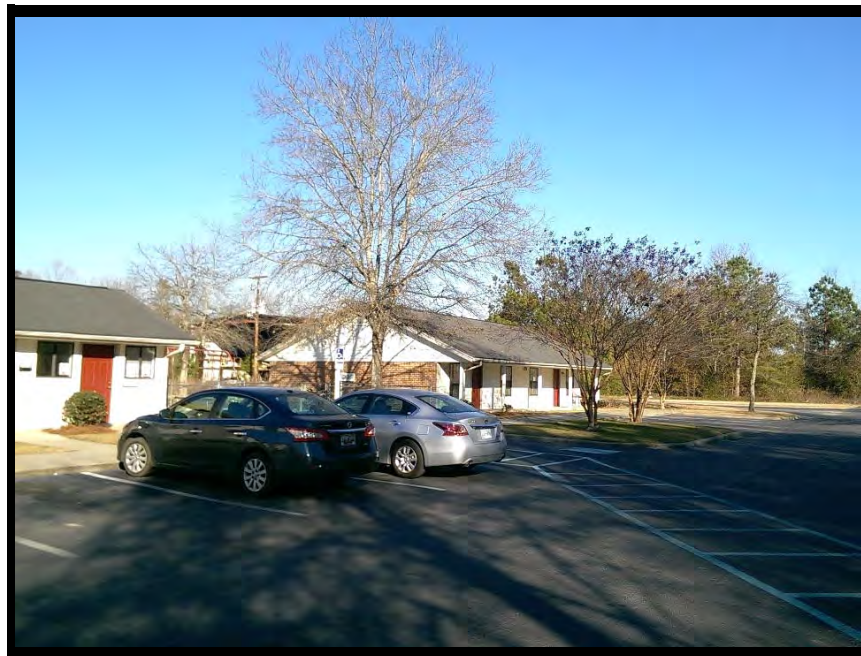
View of site from the southwest
