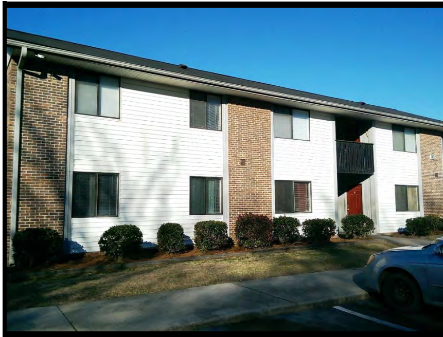
Site Phase I - Typical Building
