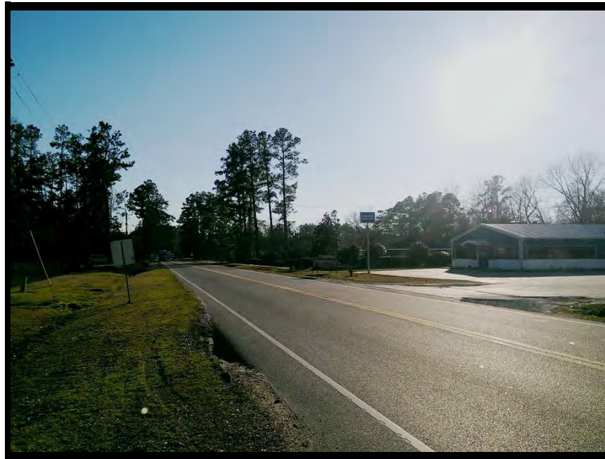
Streetscape - South View of Judge Street
